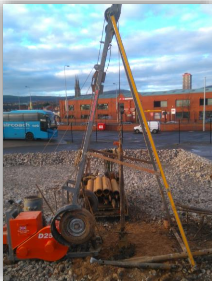
Cable percussion rig set-up in position over borehole
