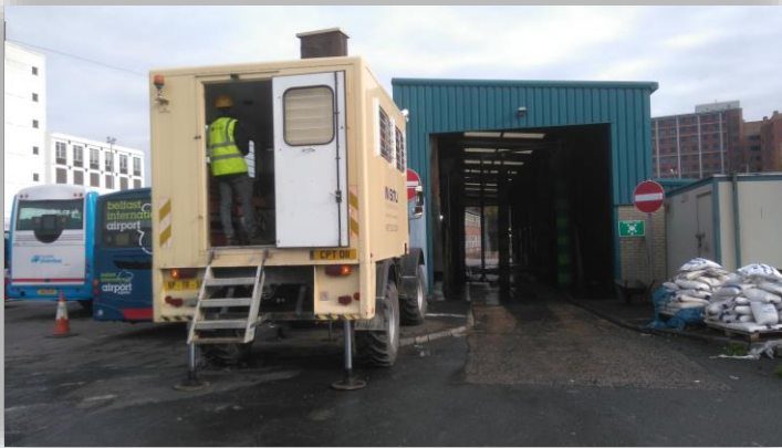
CPT works underway in Europa Bus Station
