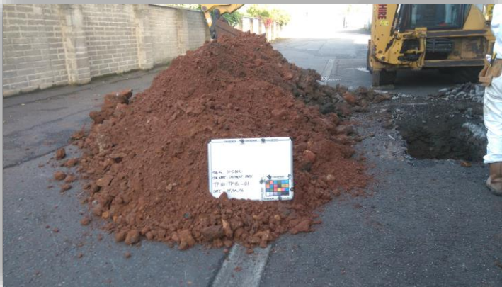
Trial pitting works underway behind the main stand
