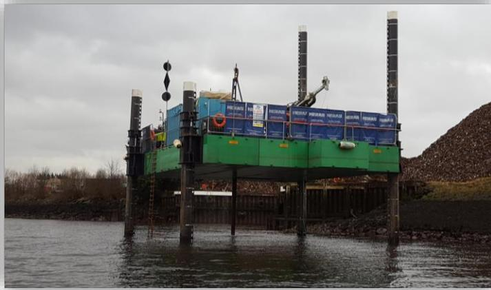
Jack-up barge set-up in position over borehole location
