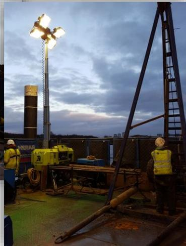
Acoustic attenuation panels and tower lights allow production through the night
