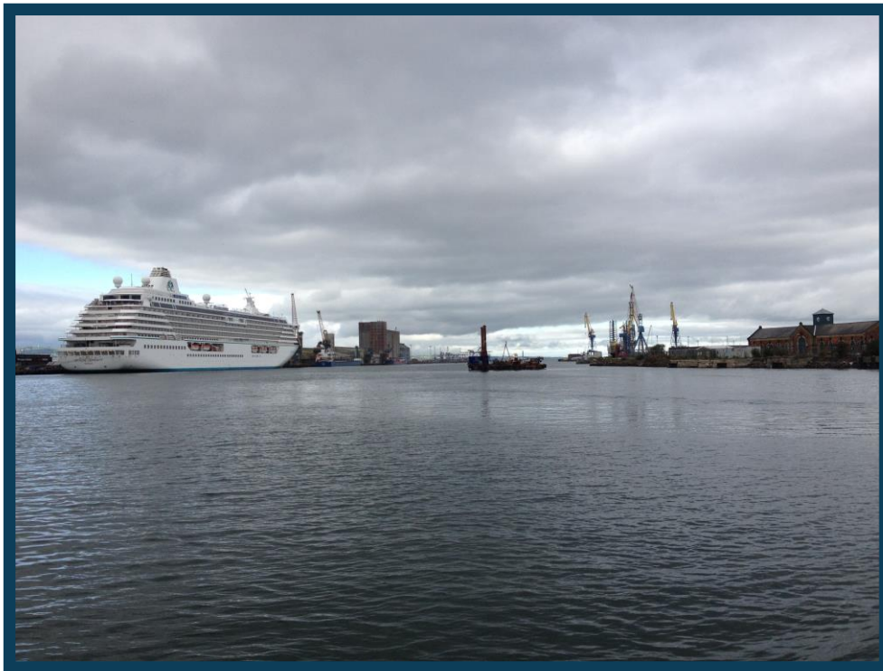
Marine spread (spud-leg barge loaded with cable percussion boring rig and rotary drilling rig) set-up over borehole location – centre of picture. Existing cruise ship terminal to left hand side of picture.
