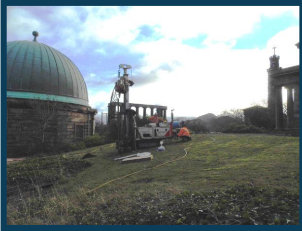
SETTING UP THE ROTARY DRILLING RIG.
