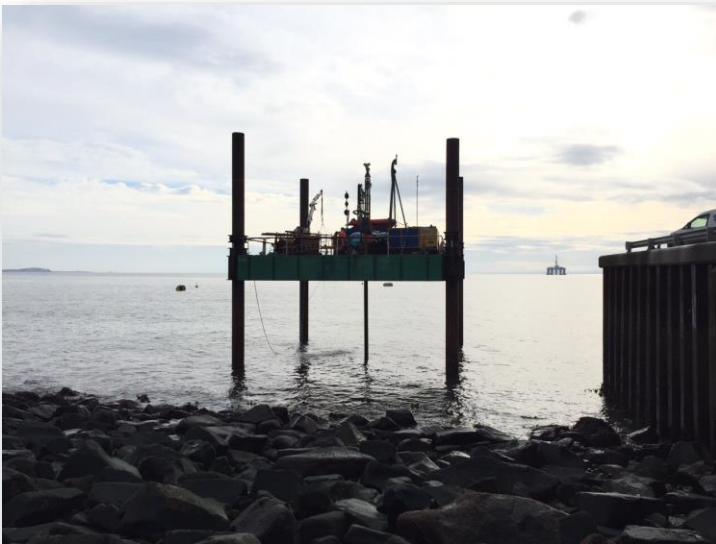
Drilling works underway at a nearshore borehole location
