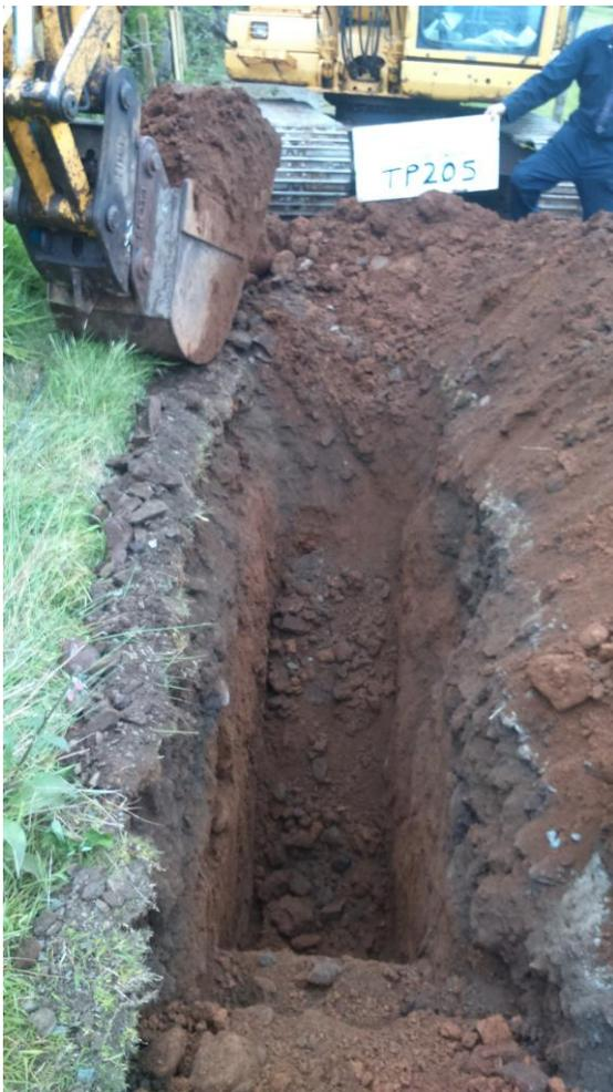
Trial pits were dug using a 13t tracked excavator with a 600mm wide bucket to depths of 1.00-3.50m.
