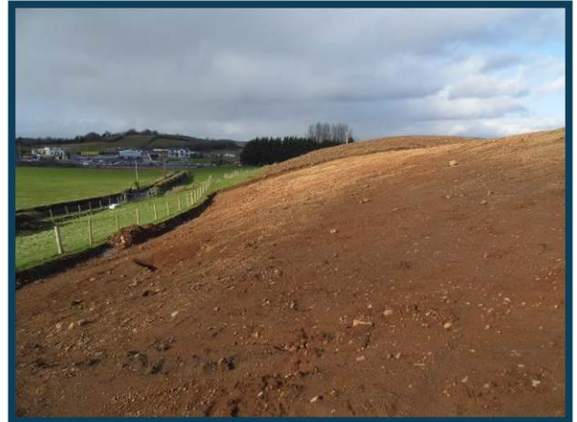
UNDULATING TERRAIN WITH TOPSOIL STRIPPED REQUIRED
