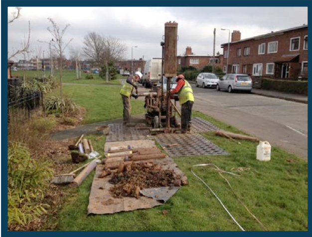
Dynamic sampling crew set up over geoenvironmental borehole location
