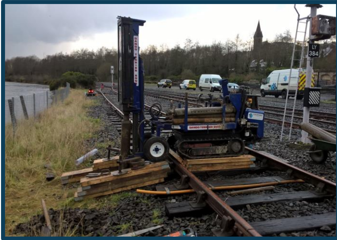
Dynamic sampling rig set up over borehole location along railway.
