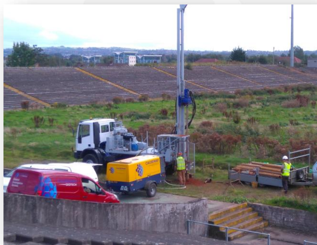
Drilling works underway at pitch side borehole location
