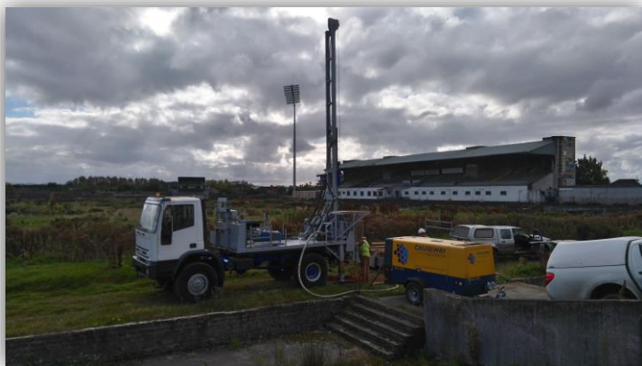
Rotary rig set-up in position over borehole location
